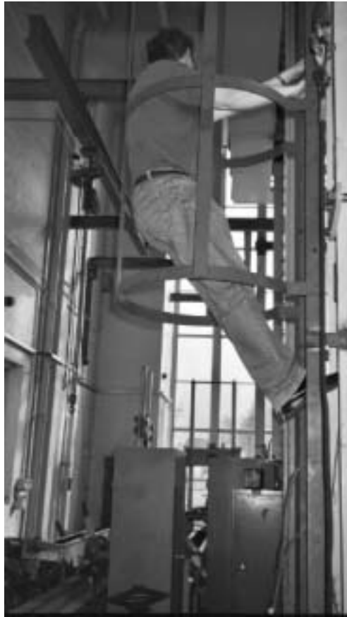
Figure 3 Climbing up caged ladder
