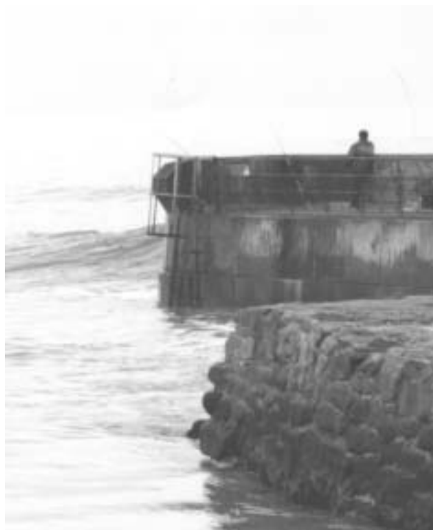
Figure 22 Caged ladder at mooring point
