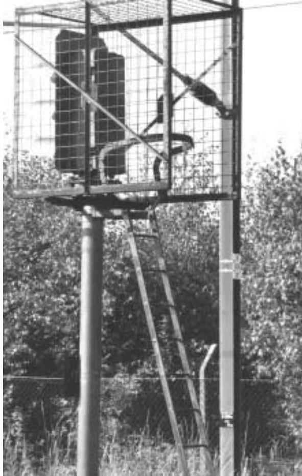
Figure 24 Single hoop formed by extension to top of ladder used for work positioning purposes
