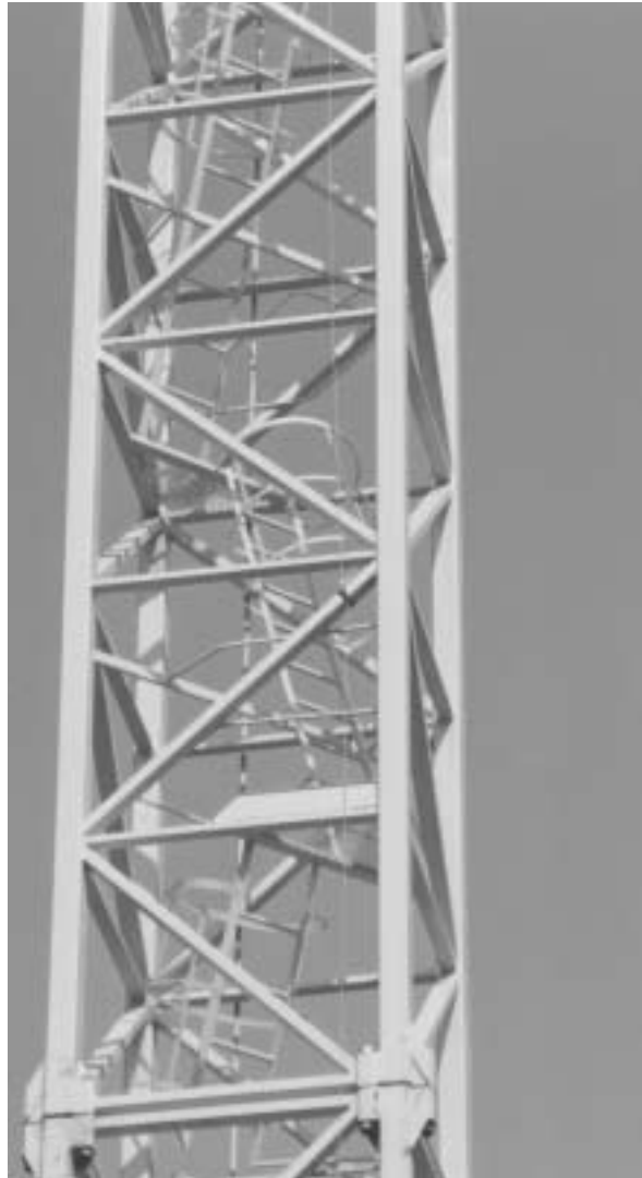
Figure 23 Caged ladder on crane tower with zigzag run
