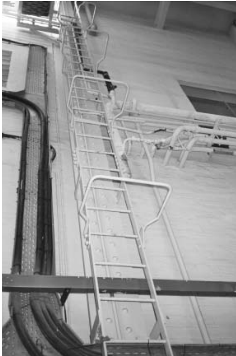
Figure 16 Safety hoops without vertical bars
